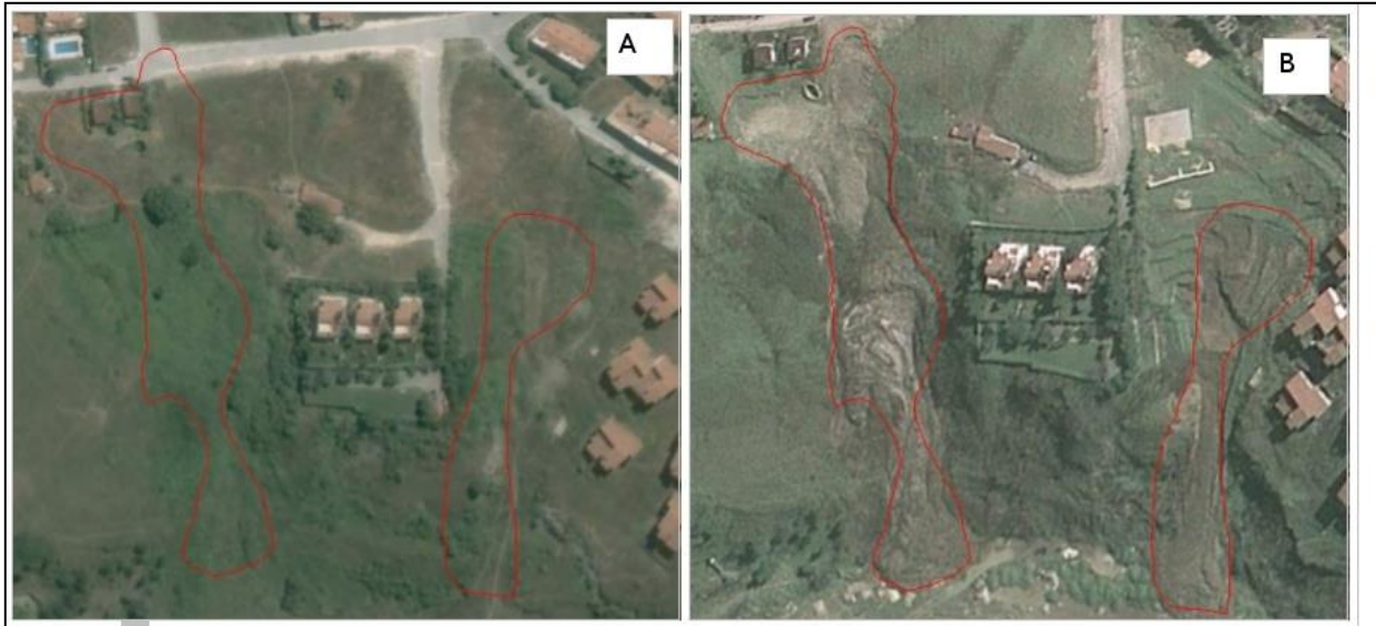
Figure 25 : Active landslide probably dated back to 2009-2010, in the western part of Avcılar peninsula detected on Google Earth Images recorded in 2004 (C -no landslide) and 2010 (B – shallow landslides).
