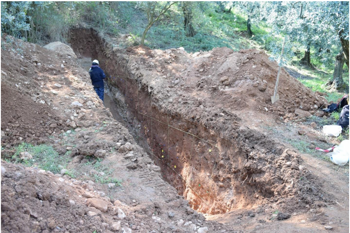
Figure 15. View of the Right bank Mustafali trench (site #3) from north.
