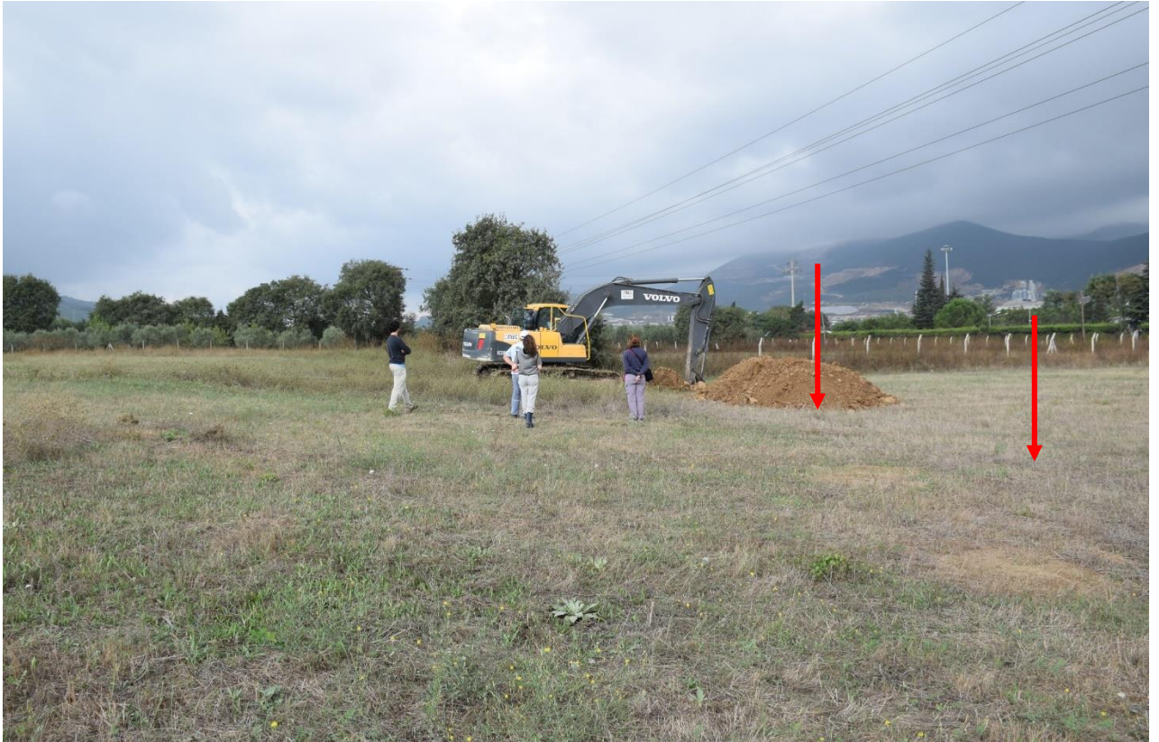
Figure 11. View of the trench site #1b. Arrows indicate the scarp base.
