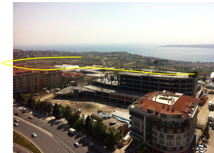
Partial overview of the Beylikdüzü landslide from the roof terrace of the shopping center.
